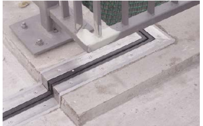
Eilenburg bridge renovation
