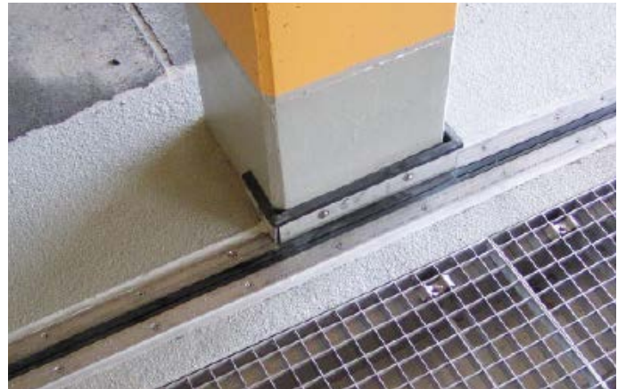
Parking deck Annaberg – FP 90
